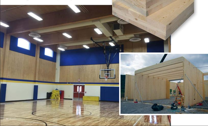
"CLT panel thickness is dependent on span and loads, so when we needed to avoid columns, we just increased the thickness of the CLT floor panels to increase the allowable spans," said Wean. "We did the same for the CLT roof panels, which ranged in thickness from about 5 to 9-9/16 inches, and were nearly 8 feet wide and 40 feet long."
