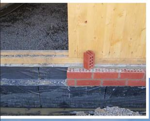
they used a vapor barrier similar to that used on any other wood-frame structure with a brick facade.
